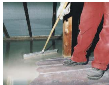
Fibre-reinforced PCI Periplan Extra is especially suitable to level wooden floors and particle boards when renovating and refurbishing.
