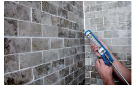
The use of PCI Carraferm prevents natural stones from staining in edge areas.
